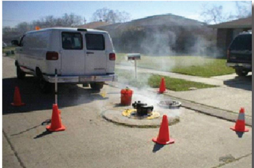
*Smoke test conducted on open manhole*
