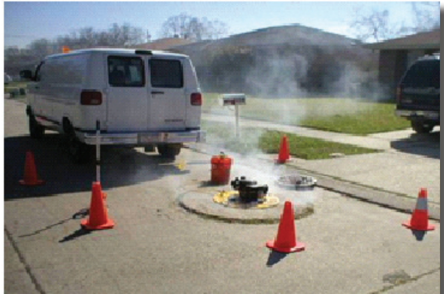
Smoke test conducted on open manhole
