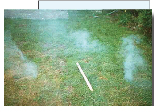
Smoke exiting the sewer system indicating defects
